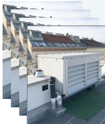
Sound insulation housing retrofitting source: kellner engineering gmbh
