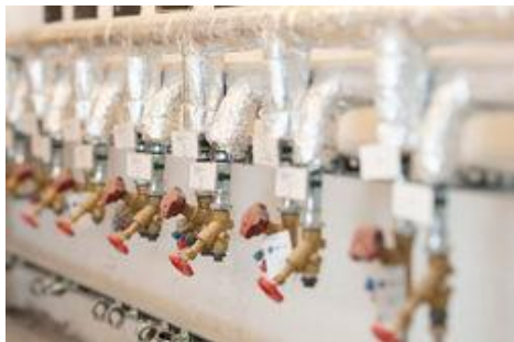
Distributor in the attic source: SOZIALBAU
