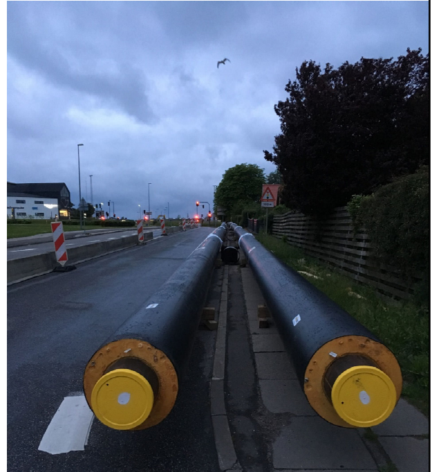
Long District Heating Pipeline without U-bends in Horsens (Denmark)
