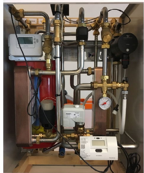
District Heating Substation with indirect connection (Alfa Laval).
