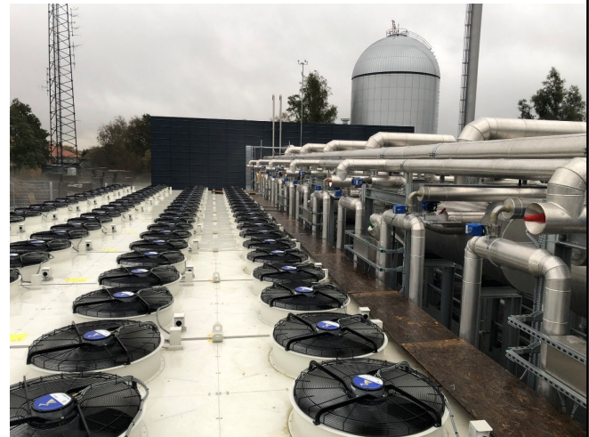
Air source for 8 MW heat pump in Støvring (DK)
